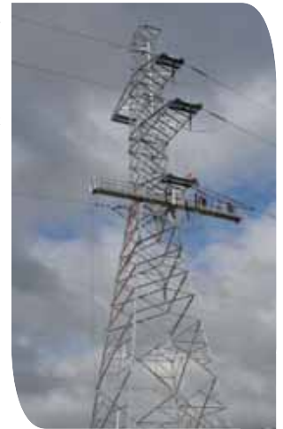
Electrix' modified strain working platform improves safety and efficiency. Linesmen can now carry out 'dead-ending' from the safety of a suspended platform that is securely anchored to the tower and ground.
