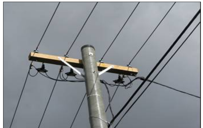
Auditing O/H construction fibreglass pole
